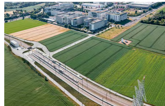
The RTW2 line connects to the RTW line in Eschborn-Ost.
