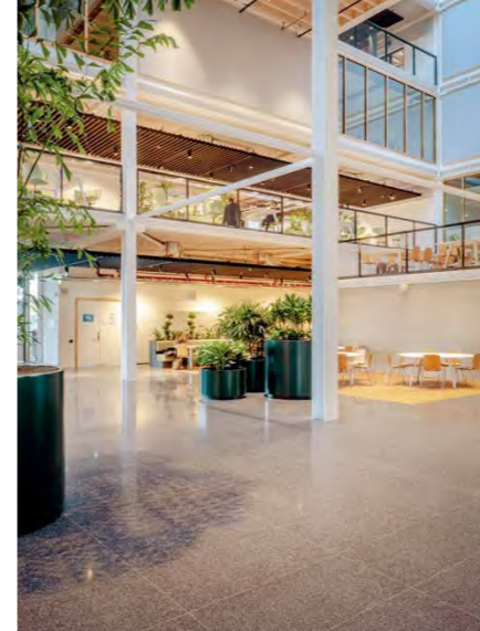
Recycled building materials and minimal material use come together in the energy-neutral building.
