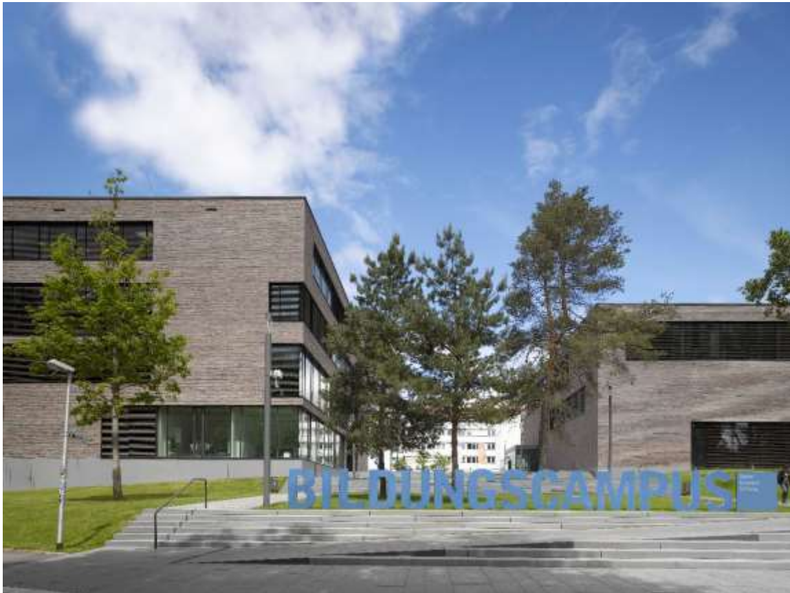
The Heilbronn Education Campus will help the city of Heilbronn achieve climate neutrality. © Roland Halbe
