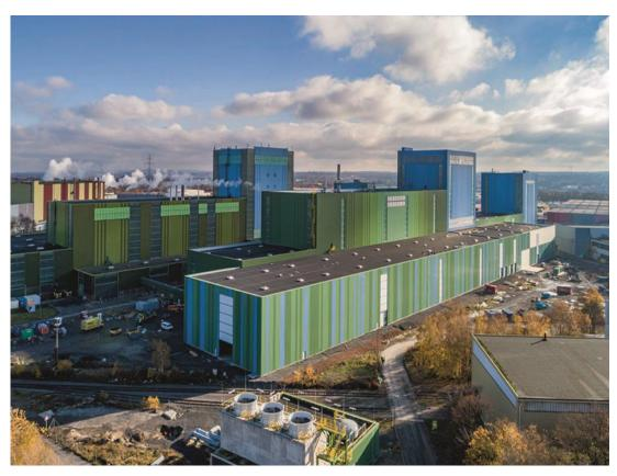
The new FBA 10 hot-dip galvanizing line at thyssenkrupp Steel in Dortmund will produce steel mainly for vehicles and household appliances on an area of around 12,600 square meters.
