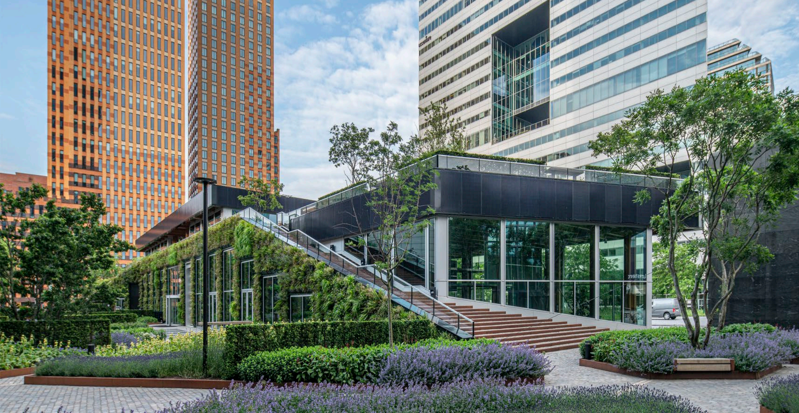
Green façade, CIRCL, ABN Amro Bank, 2014-2016. Architecten Cie. 3.350 m2
