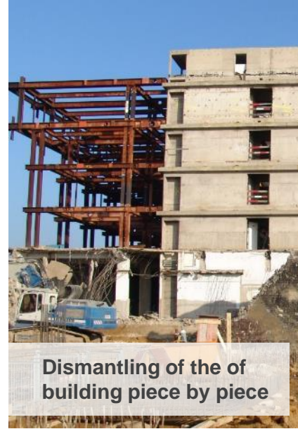
Re-conditioning and reuse of each piece in the new building
