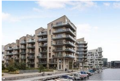
Condominium (owner-occupied housing)
