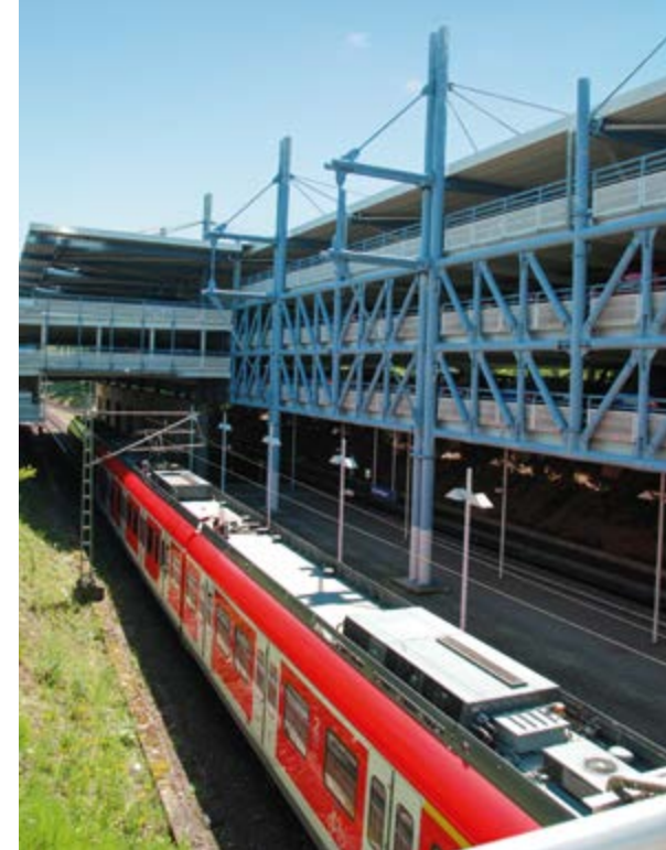
10 Park & Ride parking garages entice drivers away from their cars before they enter city center
