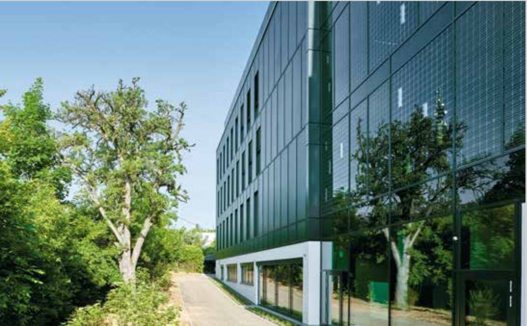
The PV facade turns OWP12 into an energy-plus building.
