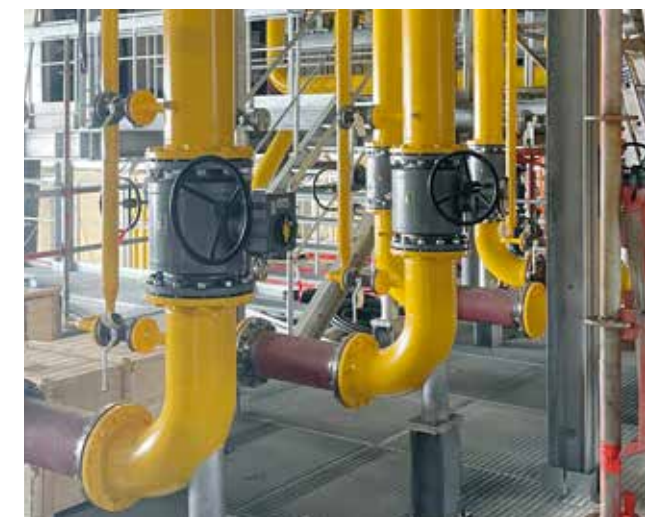
Pipe installation in the new energy center – hot water instead of steam in the „Weißenburger Straße“.
