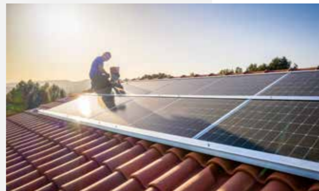
Photovoltaics on buildings
