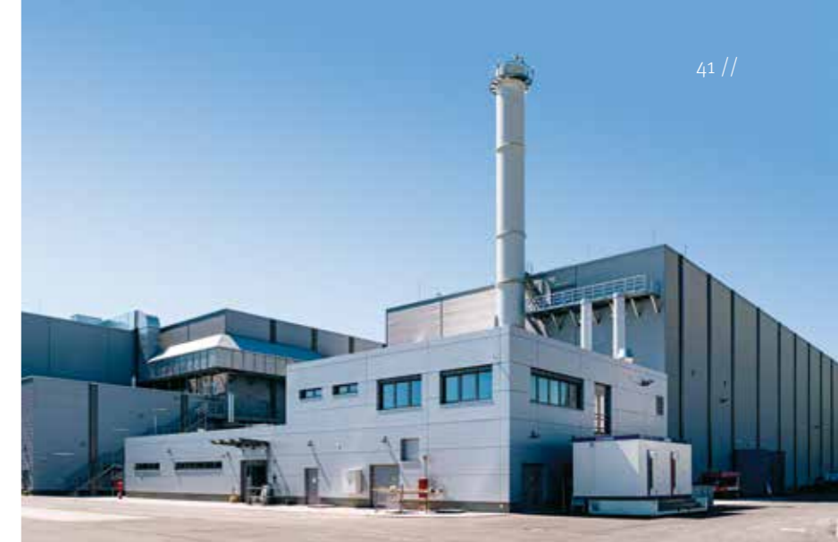
The residue processing center in Philippsburg has already been in operation since December 2020.
