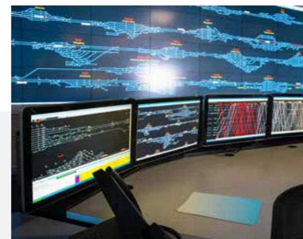
Digital train control system
