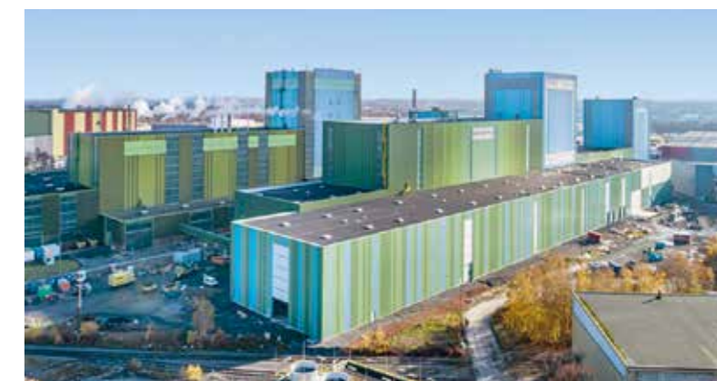
The hot-dip galvanizing line in Dortmund is 375 meters long.
