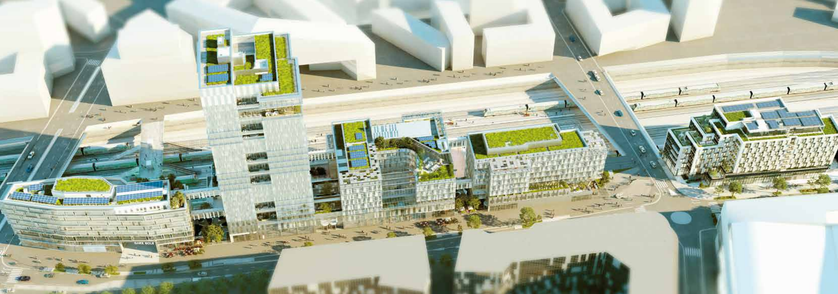
The VINCI headquarters complex L'archipel in Nanterre comprises five different buildings.
