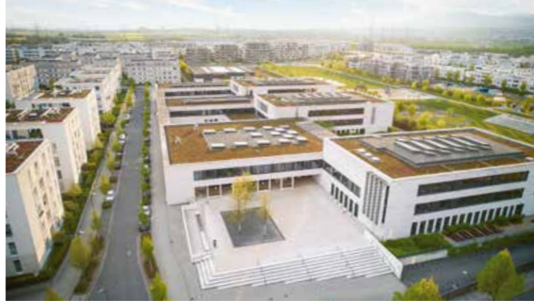
Completed in 2013, Gymnasium Riedberg grammar school's passive-house buildings offer 1,500 students a modern learning environment.
