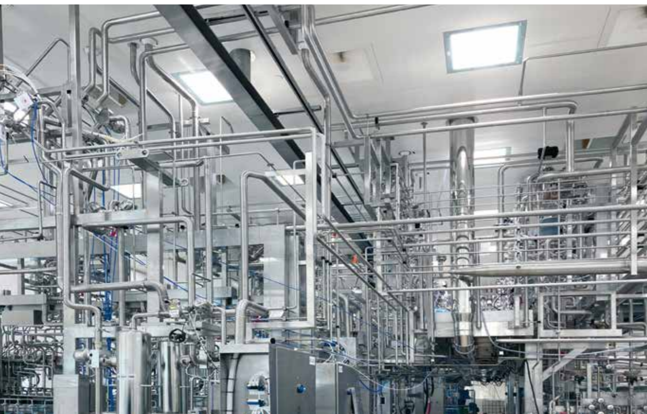
Systematic complexity: Installation of the biotechnological pharmaceuticals production facility.
